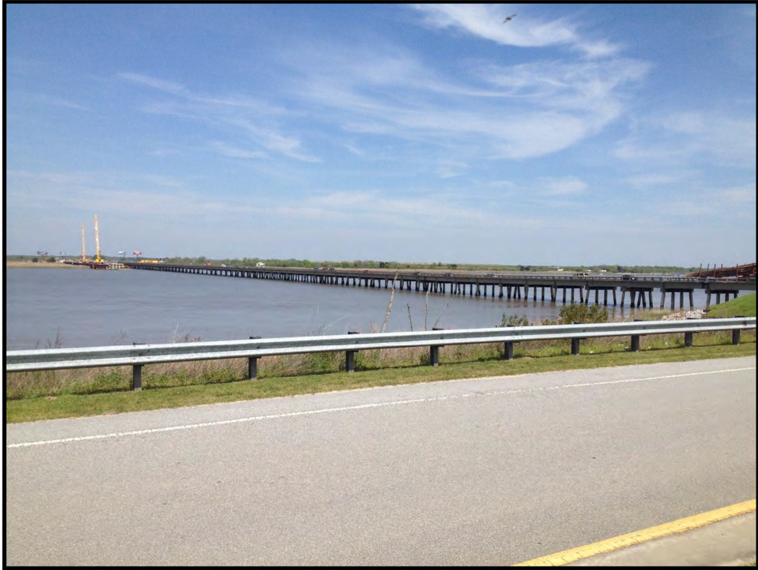
Photograph 2 – Back River on west side of U.S. Route 17
